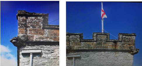
The battlements are a later addition to the tower top. There is a gutter to collect rain water from the roof so the carving to the left is not a gargoyle. The one on the right is also a hunkypunk.
