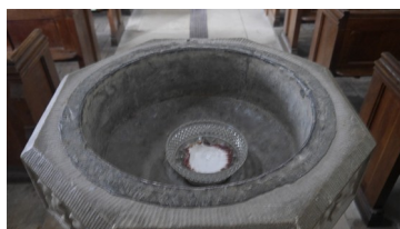
The present font with the cover removed showing the lead lined basin.
