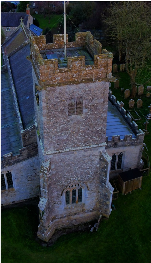
The battlements are a later addition to the tower; date unknown.
